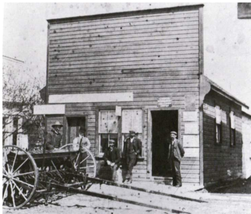
The premises of Harrower and Price which doubled as the Municipal Office.
